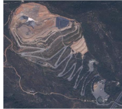
Construction and exploitation of Phase 2 of the current authorization (extends until 2026) at the Bossarino landfill .
