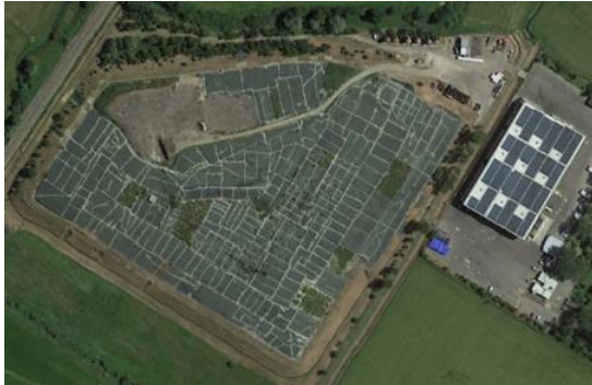
Expansion of the Albonese landfill with the creation of a new reservoir for approximately 450,000 additional cubic meters.
