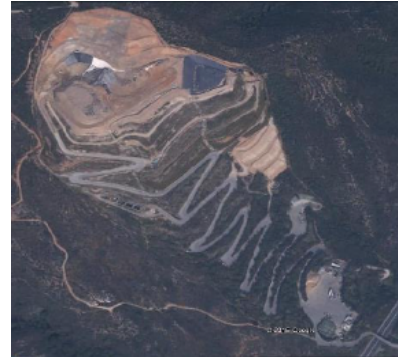
Construction and exploitation of Phase 2 of the current authorization (extends until 2026) at the Bossarino landfill .
